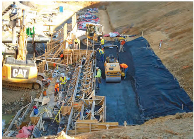
FIGURE 9-13. Hand placement of RCC.
