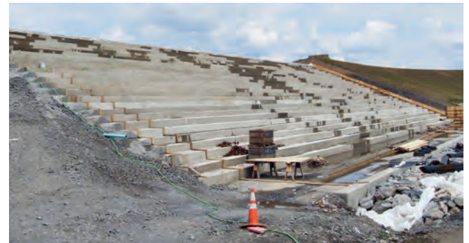
FIGURE 6-12. Formed RCC chute (Toby Creek Impounding Basin, PA), courtesy of KC Construction.
