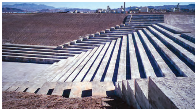
FIGURE 6-42. Formed sloped RCC training walls with deflection blocks to prevent erosion (Anthem Dam, NV).
