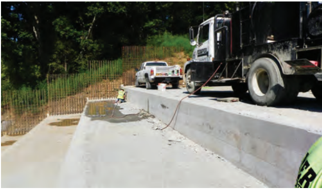
FIGURE 6-13. Formed grout enriched RCC steps.
