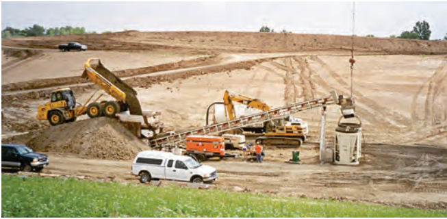
FIGURE 9-10. RCC loaded into concrete bucket to be delivered to placement area via crane.
