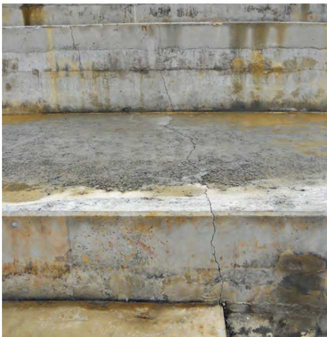
FIGURE 6-34. Naturally occurring shrinkage crack in RCC.
