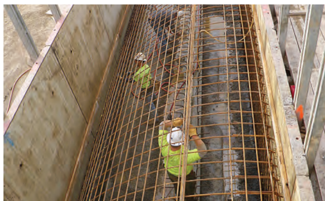
FIGURE 6-21. Top view of installation of reinforcement for ogee crest weir (Fox Creek MPS No. 4, KY).
