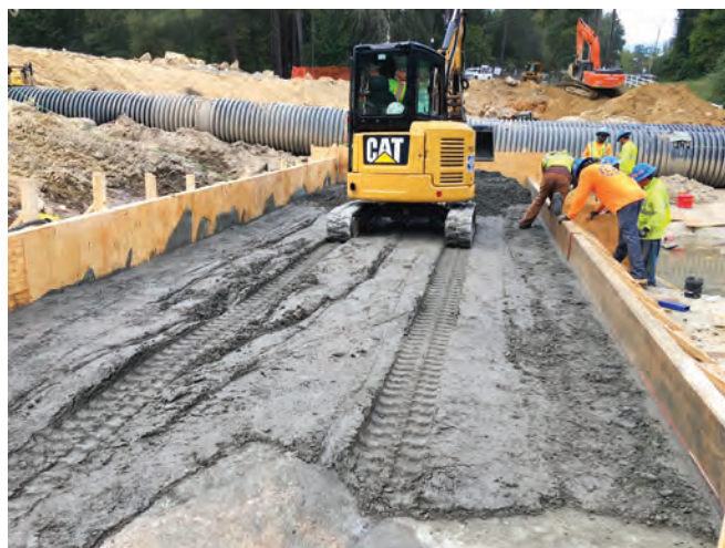
FIGURE 7-3. Typical fresh IVRCC surface.
