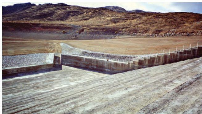
FIGURE 6-44. Vertically formed RCC training walls (Red Rock Canyon Detention Dam, NV).
