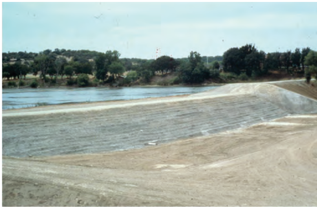
FIGURE 9-19. Unformed, uncompacted RCC steps.
