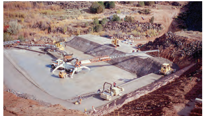
FIGURE 9-9. “Super Swinger” conveyor delivery system.
