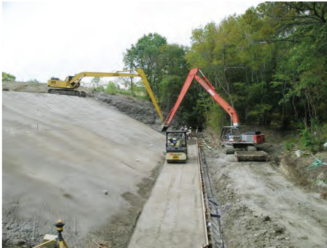
FIGURE 9-7. RCC delivery with long stick hydraulic excavators.
