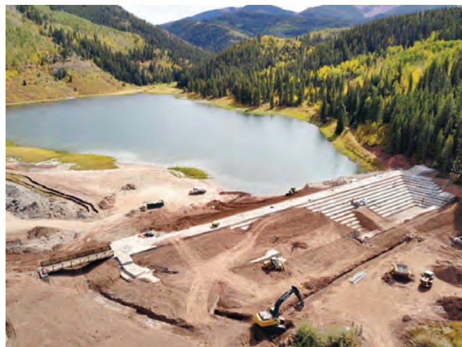
FIGURE 6-50. RCC spillway with topsoil cover placement in progress (Sylvan Lake Dam, CO).
