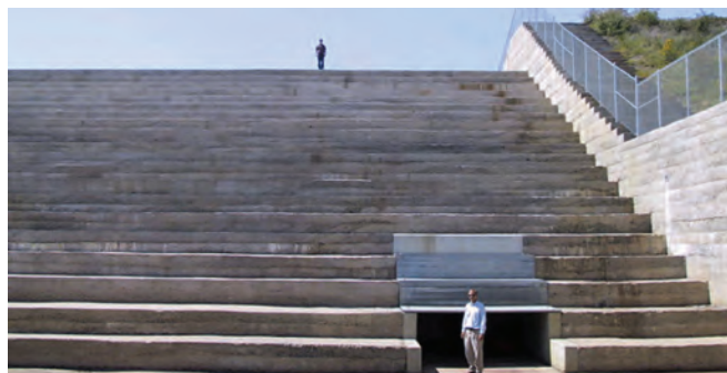
FIGURE 6-43. Vertically formed RCC training walls (East Fork Above Lavon 3C, TX), courtesy of Dennis Clute.
