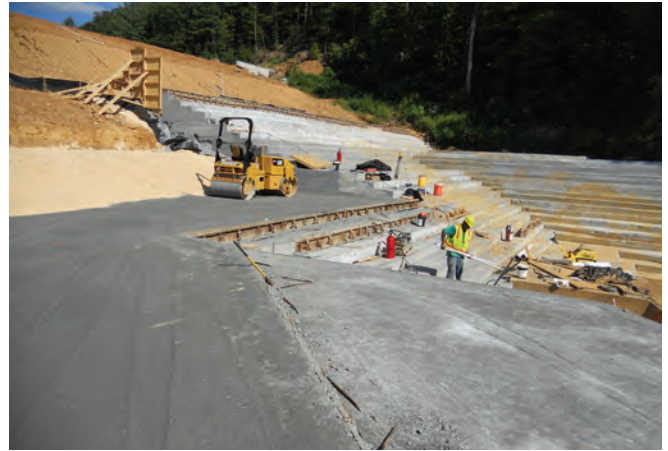
FIGURE 9-31. Placement of RCC at transition area.
