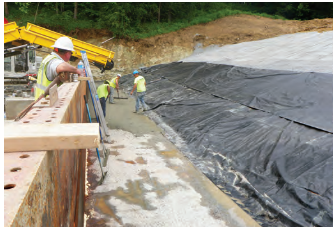
FIGURE 9-30. Bedding mortar placement.
