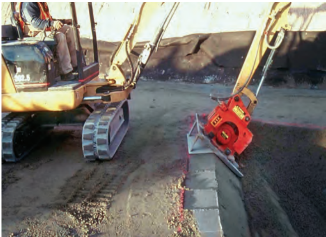
FIGURE 9-17. Vibratory plate compactor attachment on hydraulic excavator used to compact exposed RCC face.
