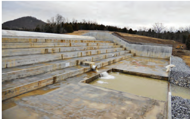
FIGURE 6-27. Run-out apron, end sill and riprap transition (Fox Creek MPS No. 4, KY).
