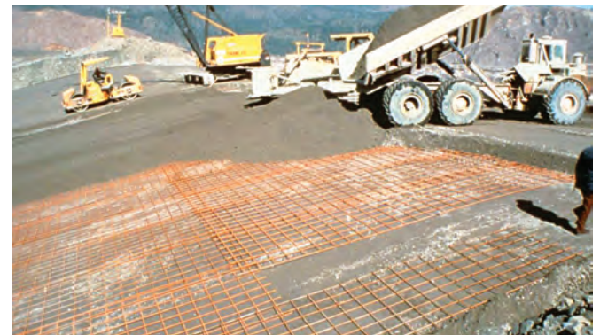
FIGURE 6-5. RCC plated spillway (Toutle River Dam, OR).
