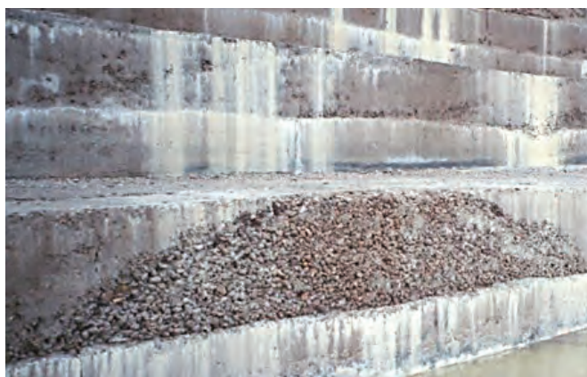
FIGURE 9-23. Poor RCC face.
