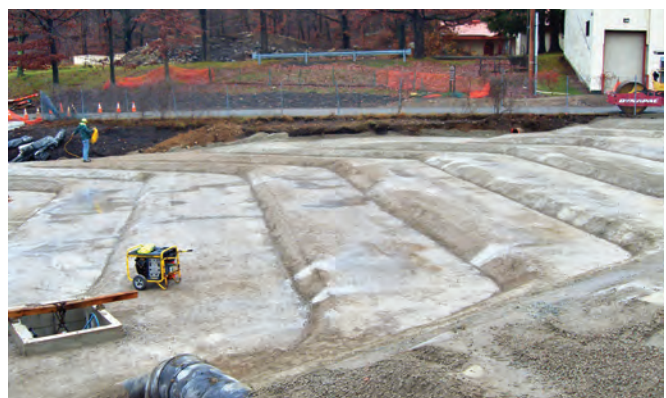
FIGURE 6-10. Unformed RCC chute with compacted RCC (Picati Lake Dam, NJ), courtesy of KC Construction.
