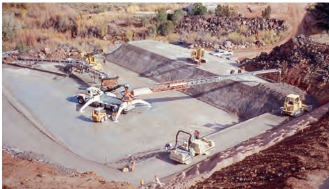
FIGURE 6-25. RCC spillway prior to installation of fuse gates shown in Figure 6-24 (Black Rock Dam, NM).
