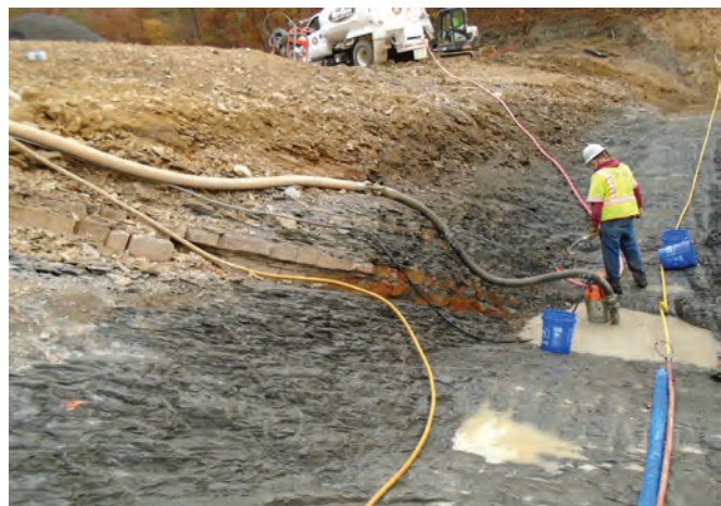
FIGURE 9-1. Dewatering sump adjacent to downstream cut-off wall in stilling basin runout apron.
