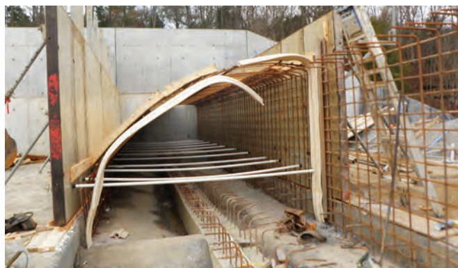
FIGURE 6-20. Side view of installation of reinforcement for ogee crest weir (Fox Creek MPS No.4, KY).
