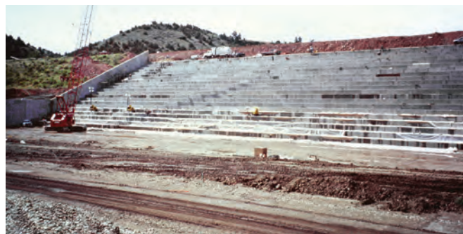
FIGURE 9-24. Precast CVC panels used for vertical step faces (Tongue River Dam, MT).
