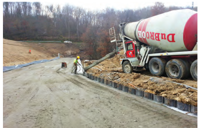
FIGURE 6-32. Backfilling steel sheet pile cutoff with conventional concrete (Lake Oneida Dam, PA).
