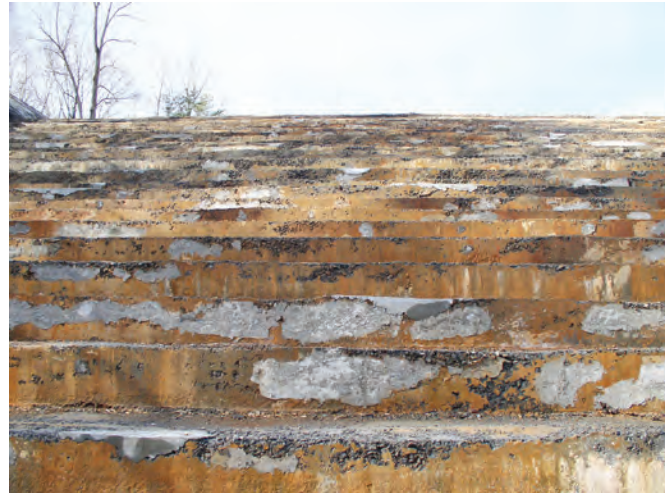
FIGURE 10-9. Damaged and poorly-patched RCC surface.
