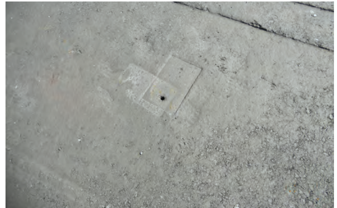
FIGURE 9-18. Typical good-quality RCC surface texture.
