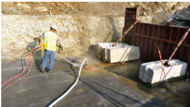
FIGURE 9-28. Preparation of cold joint.
