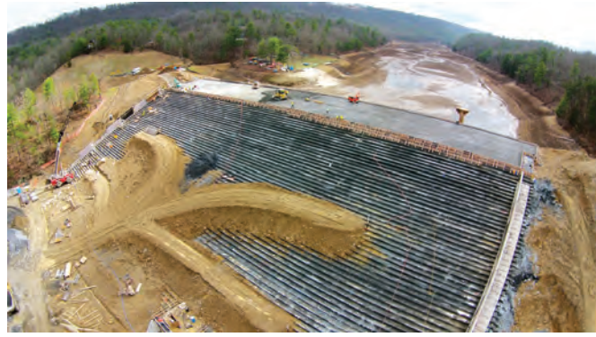
FIGURE 6-49A. RCC spillway before topsoil cover is placed (Lake Laura Dam, VA).
