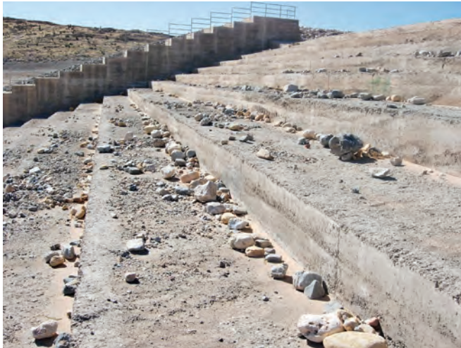
FIGURE 10-7. Debris on steps after flood event with very little loss of RCC material (Red Rock Basin, NV).
