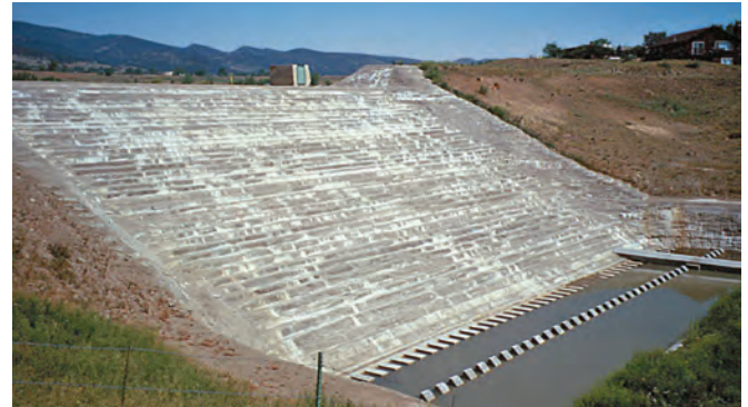
FIGURE 9-20. Unformed, compacted RCC steps.
